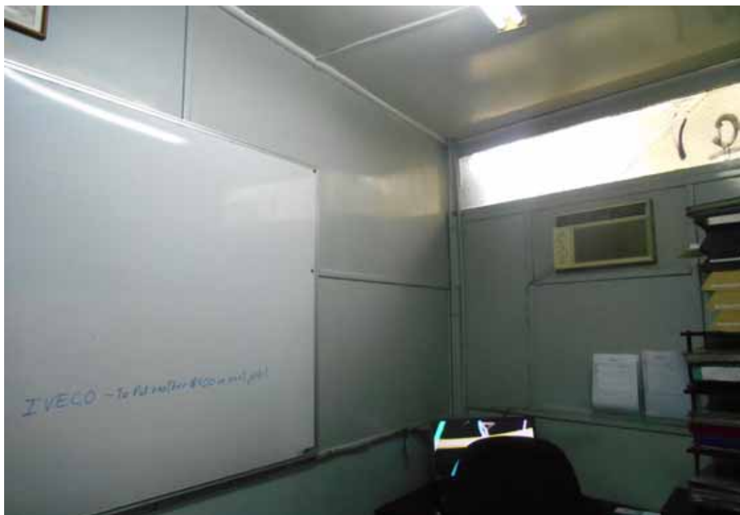
Photo 7 - Office area within workshop with FCS walls
