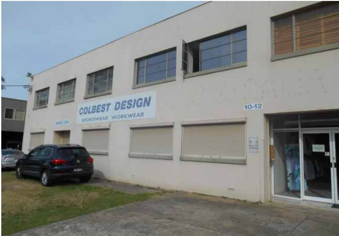
Photo 1 - Front view of 10 - 12 East Street
