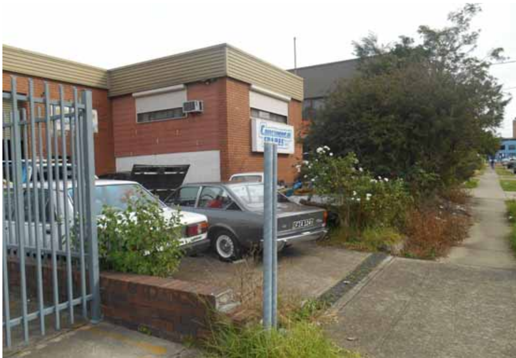
Photo 15 - Front view of 26 East Street
