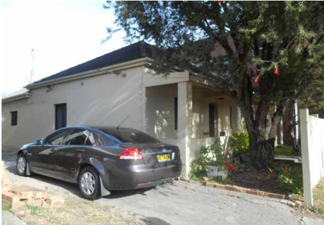
Photo 35 - Front view of 42 East Street
