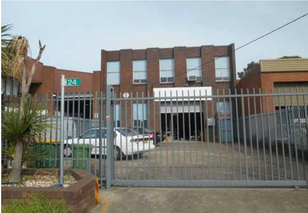
Photo 11 - Front view of 24 East Street
