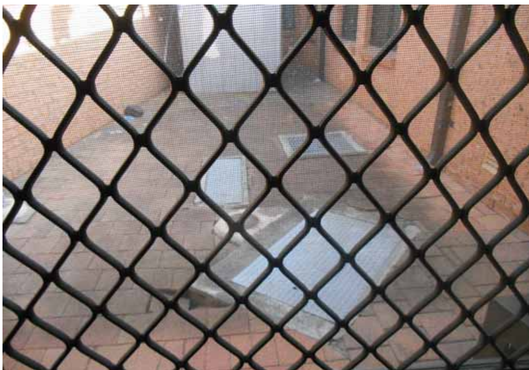
Photo 30 - Drains in western courtyard
