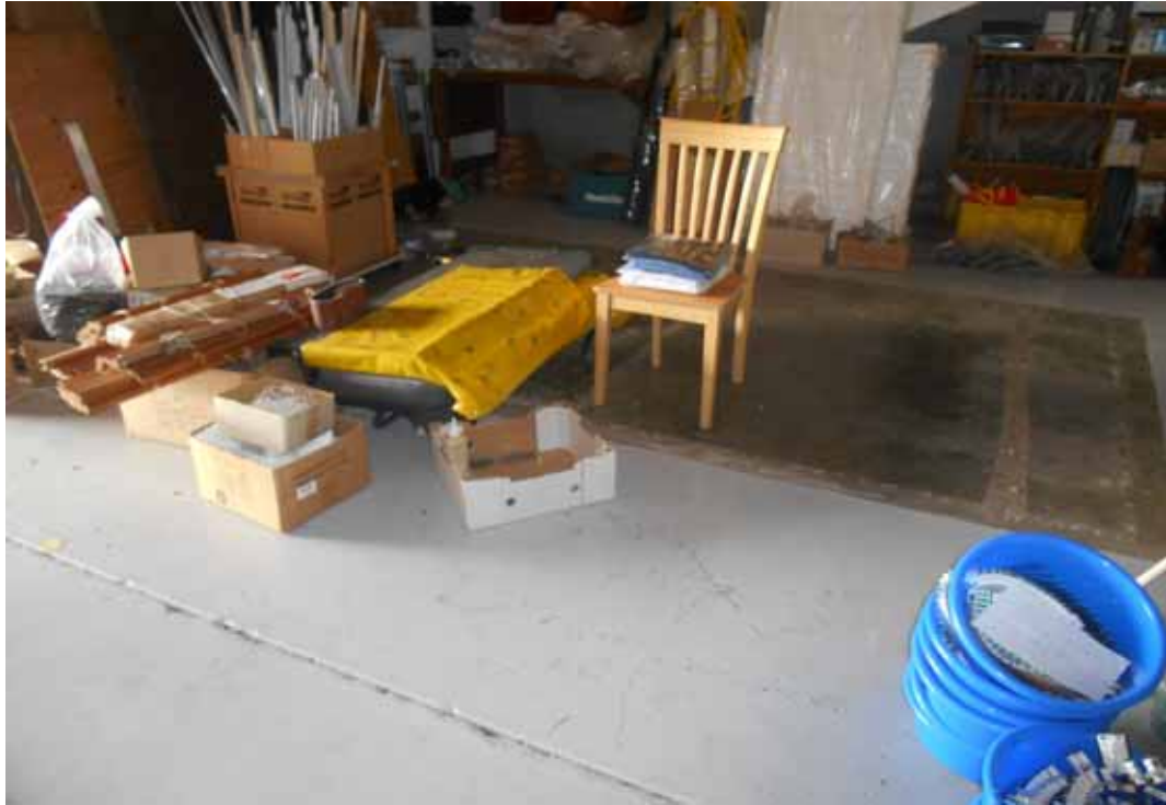
Photo 13 - Unusual square area of replaced concrete
