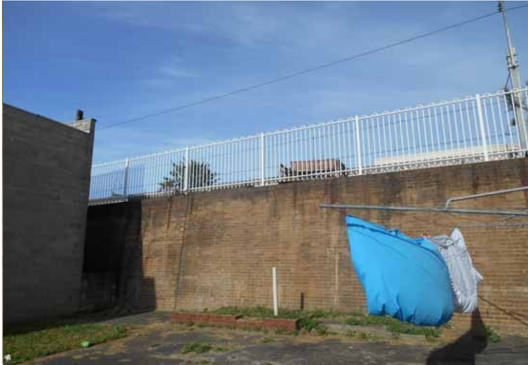
Photo 37 - Looking west towards the railway line at 42 East Street onto the retaining wall
