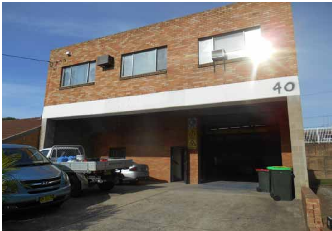
Photo 32 - Front view of 40 East Street
