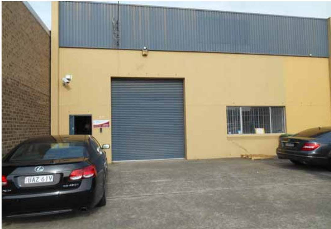
Photo 26 - Front view of 32 East Street
