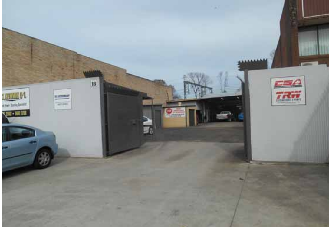
Photo 3 - Front view of 16 East Street
