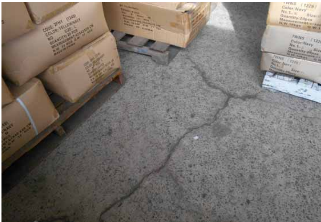
Photo 2 - Concrete in external storage area of 10 - 21 East Street
