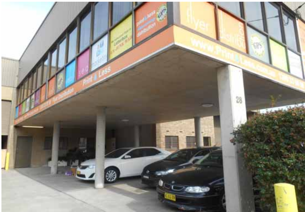
Photo 19 - Front view of 28 East Street
