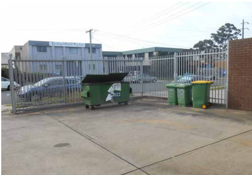
Photo 10 - Exterior hardstand of 18 East Street with minor staining of concrete observed
