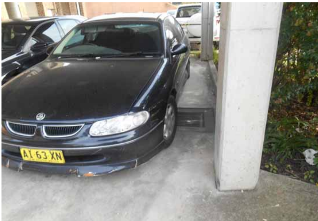
Photo 21 - Stormwater drain located in car park area of 28 East Street
