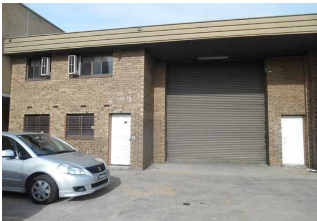
Photo 22 - Front view of 30 East Street
